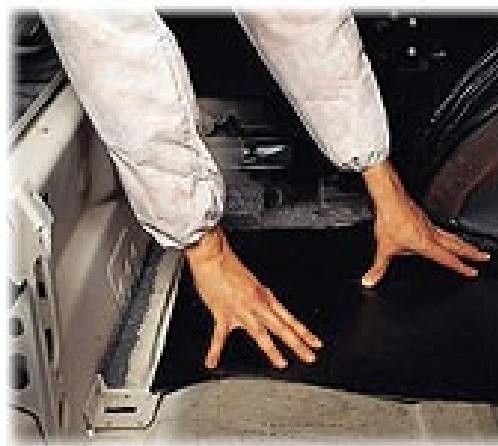
Figure 4. Installation of chosen damping material
