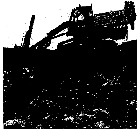
Figure 2. A Ranger drilling machine
